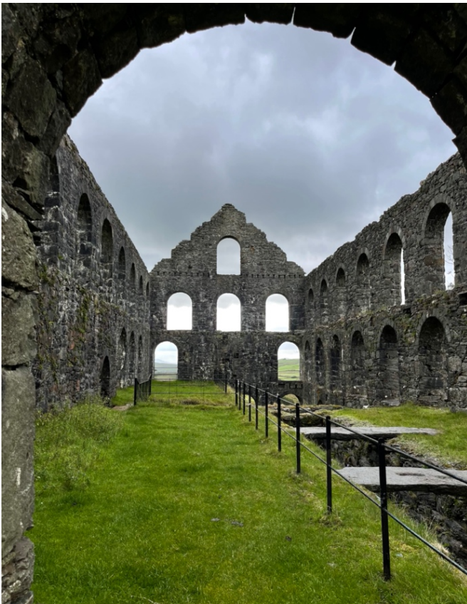
Figure 4: Photograph of the Ynys y Pandy Slate Mill’s entrance (Own Photography, 2024).
