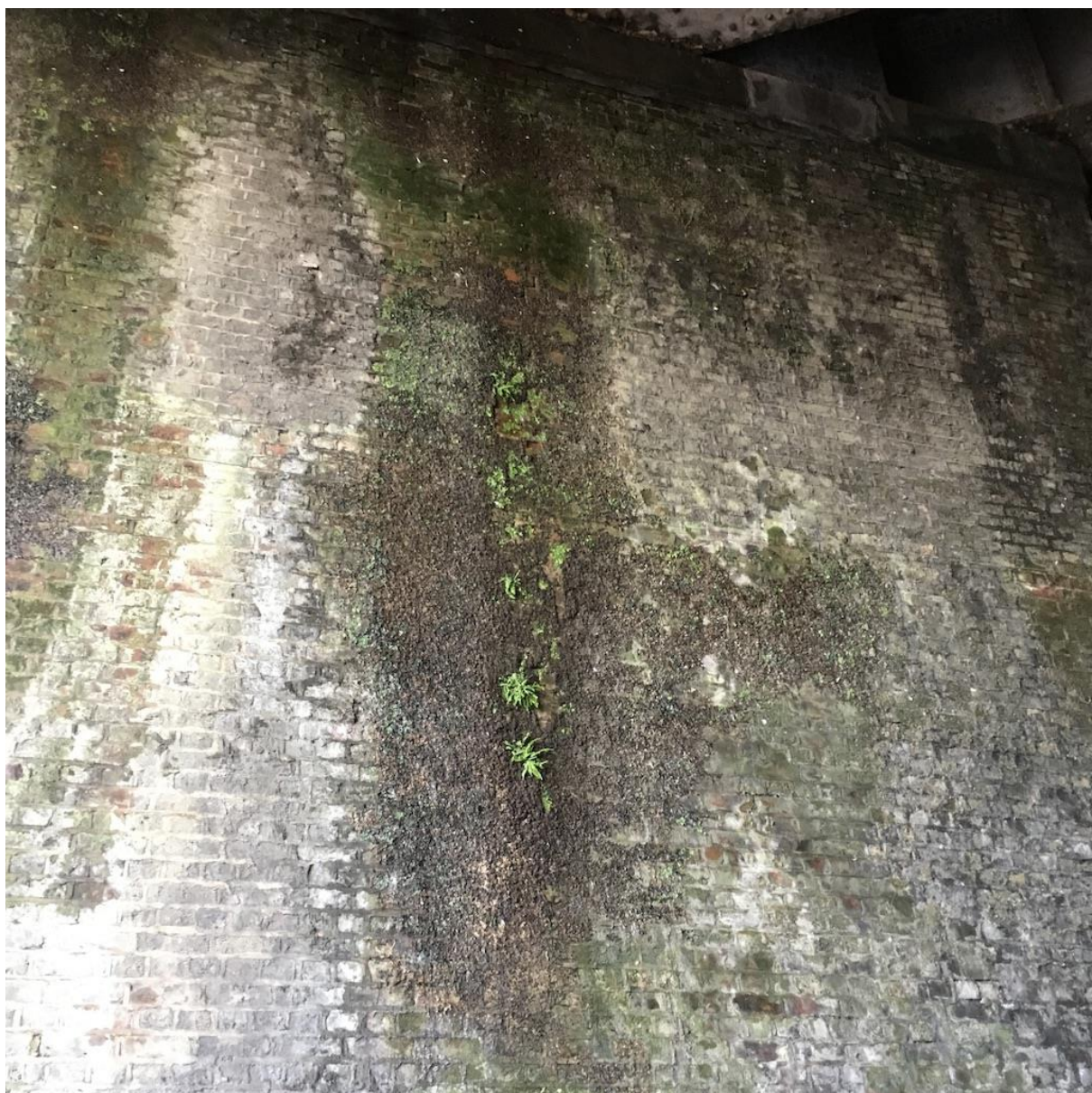
Figure 24 – Hart's tongue fern growing out of the damp wall.
