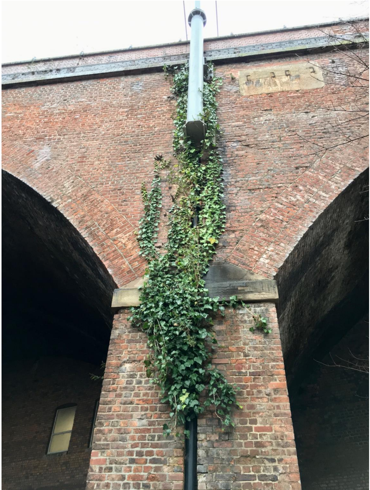
Figure 14 – ivy climbing a leaking drainpipe.
